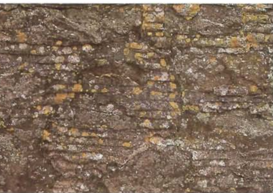
Above: Walls in Leigh pointed with Portland cement mortar turn black with time, obliterating the colour and charm of the building stone.
